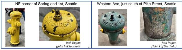
The earliest List 90s have cast on the barrel the company name as "Rensselaer Mfg.", the patent numbers, and "The Corey" on the bonnet, as seen at <a href="http://www.firehydrant.org/pictures/ren01.html">http://www.firehydrant.org/pictures/ren01.html</a>.
