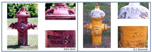
After Rensselaer became part of Ludlow-Rensselaer, hydrants manufactured by the company were cast with "Ludlow-Rensselaer."
